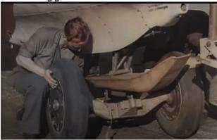
However, the skid was held in place by an oleo-pneumatic strut that absorbs the shock in landings. If this were to malfunction, the pilot was in for a very rough landing. In fact, three of its main test pilots experienced this malfunction and were hospitalized with serious spinal damage and skull fractures.
